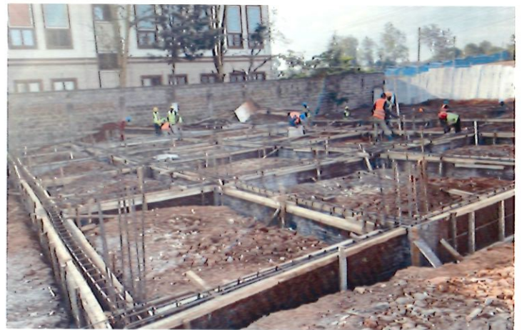
September 2024, Foundation work for the new facilities to house Runda Baptist Church.
