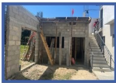
Kitchen between church on left and school on right.
